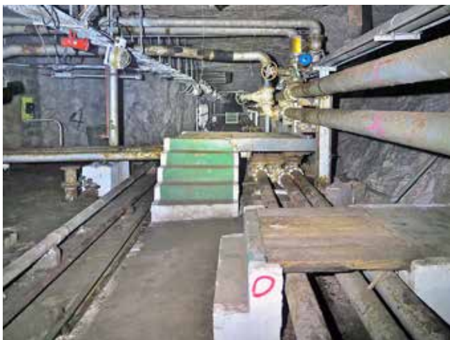
Project C: the plumbing. Photo Clive Penfold
